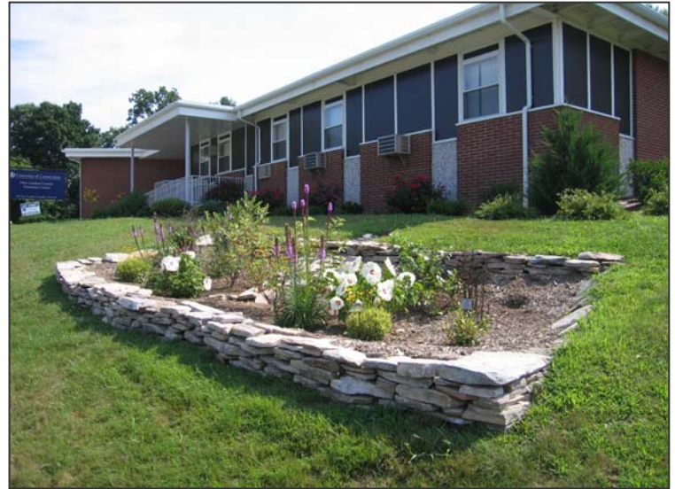
Demonstration rain garden at the New London County Extension Office in Norwich, CT
