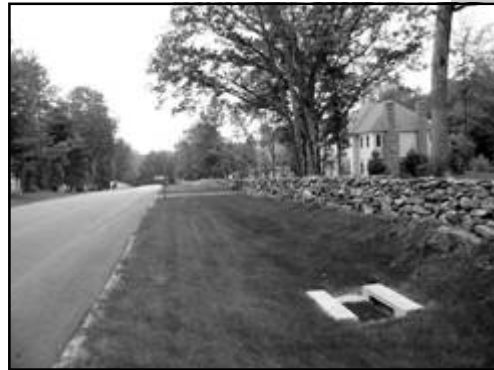
Permeable driveways and grass swales are two alternative practices that reduce runoff by encouraging infiltration.
