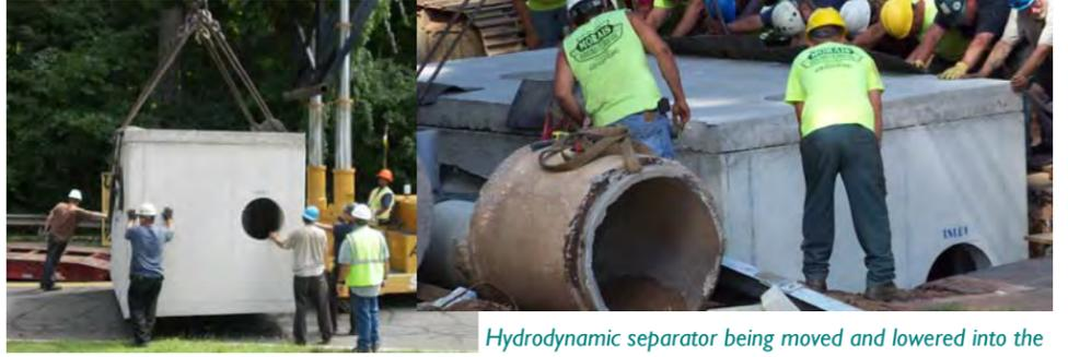
Hydrodynamic separator being moved and lowered into the ground within the roadway on Adams Street, Manchester.
